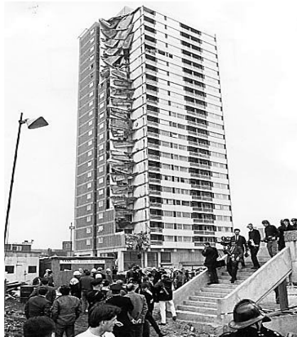
Figure 1.1 Partial collapse of Ronan Point apartment building
