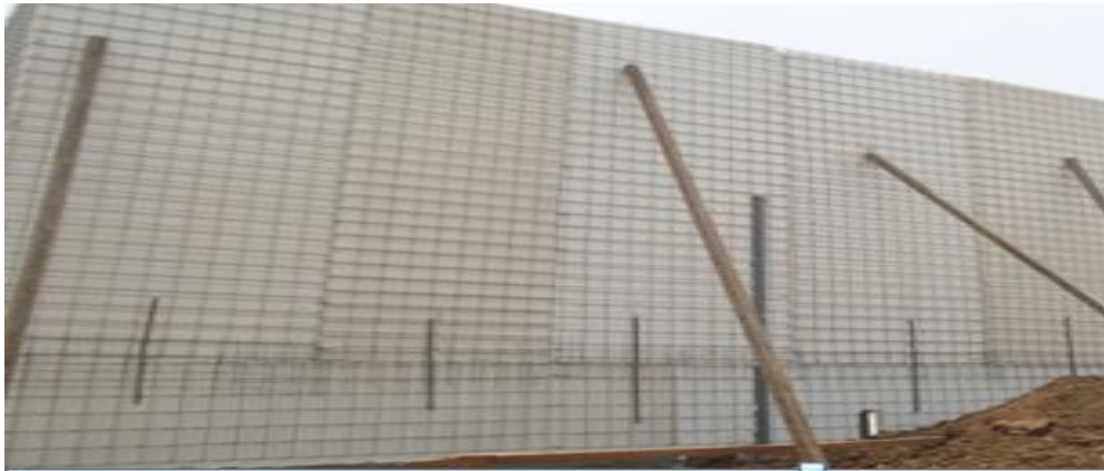
Figure 6: Polystyrene meshed panels used as wall panels on a building site in Maitama, Abuja
