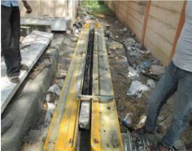
Fig.1 Steel reinforcement placed in the mould
