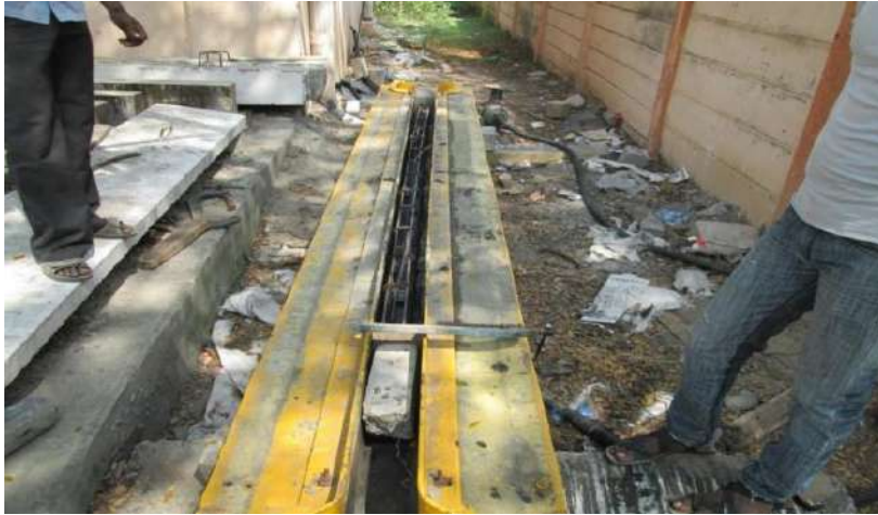
Fig.1 Steel reinforcement placed in the mould
